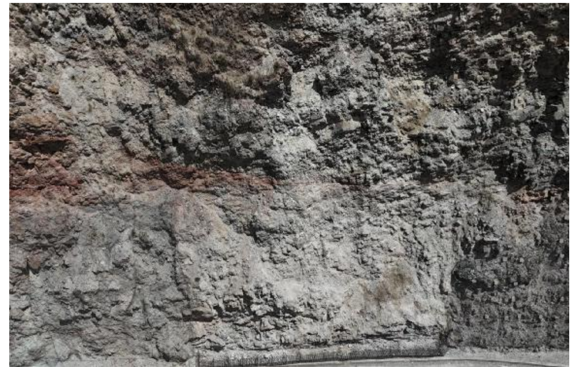
K745+621~K745+709 段左侧坡面现状
